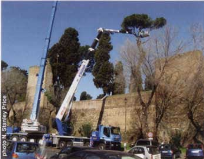
Removal of pine tree from Zona Vecchia.
